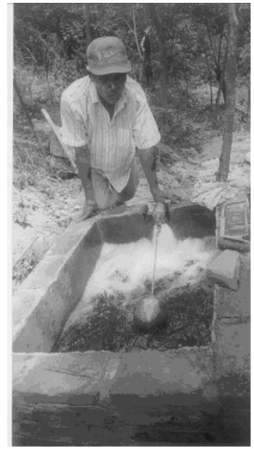
Figure 6.11 Break-Pressure Tank with Float Valve in Honduras (Simpson 2002)
