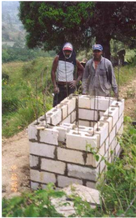
Figure 6.10 Break-Pressure Tank Under Construction in the Dominican Republic (Niskanen 2003)
