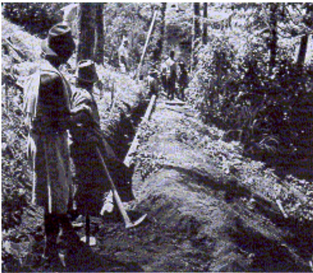
Figure 6.1 Pipeline Excavation in Kenya (IRC 1981)
